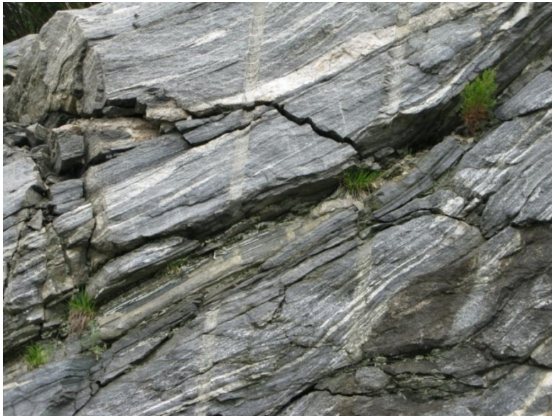
Figure 13. Offset drill-hole scars in Rope Ferry Gneiss, Rte. 11, east side of highway.
